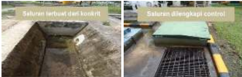
Gambar 4. Saluran Drainase Terpisah dan Tertutup ( closed system )
